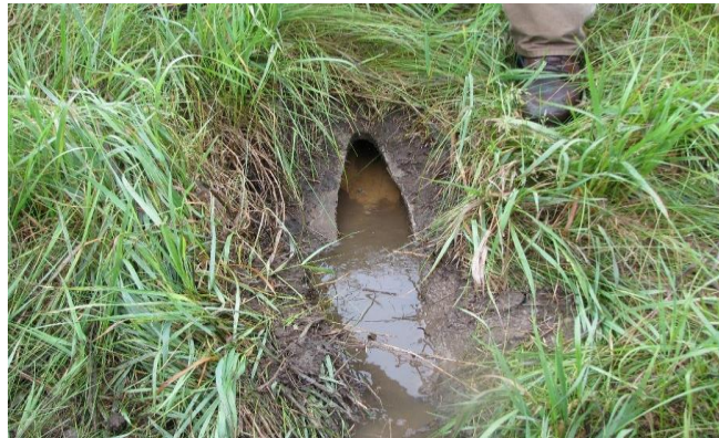
Figure 11: Plugged edge drain near surveyed Michigan sections
