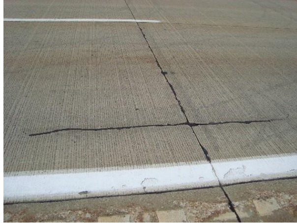
Figure 12: Longitudinal (or diagonal) cracking in the wheel path in sections surveyed in Michigan
