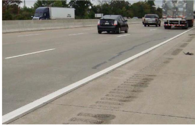
Figure 10: Longitudinal cracking due to erosion of the HMA interlayer in surveyed Michigan sections
