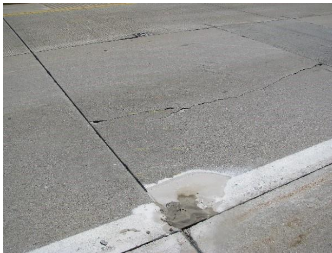
Figure 13: Midslab longitudinal cracking in surveyed Michigan sections
