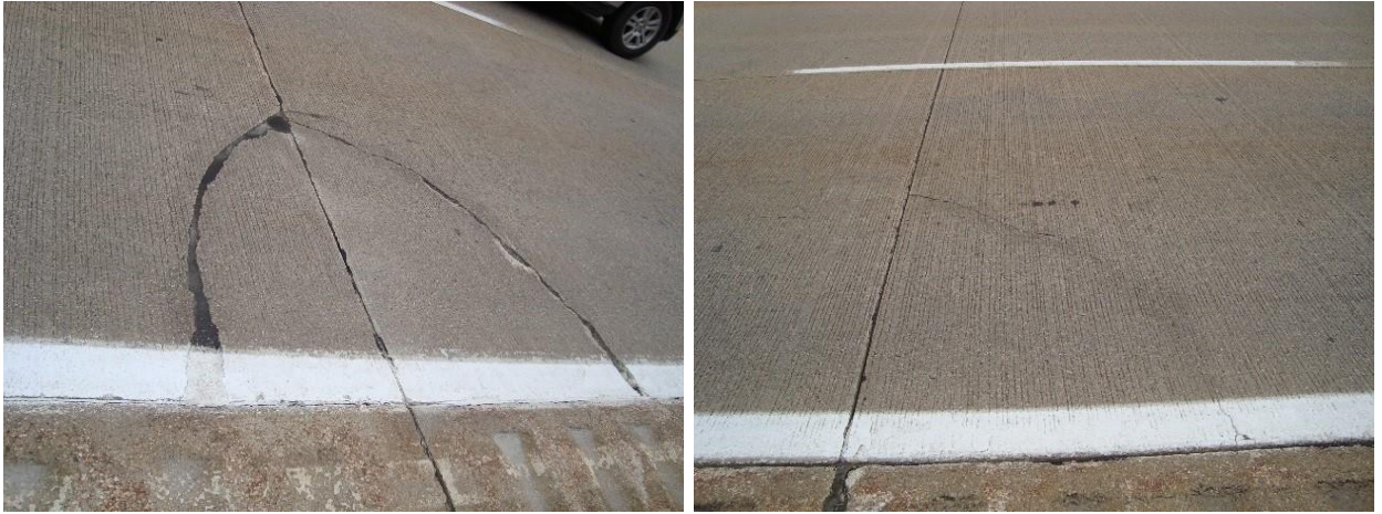
Figure 15: Corner breaks observed in Michigan
